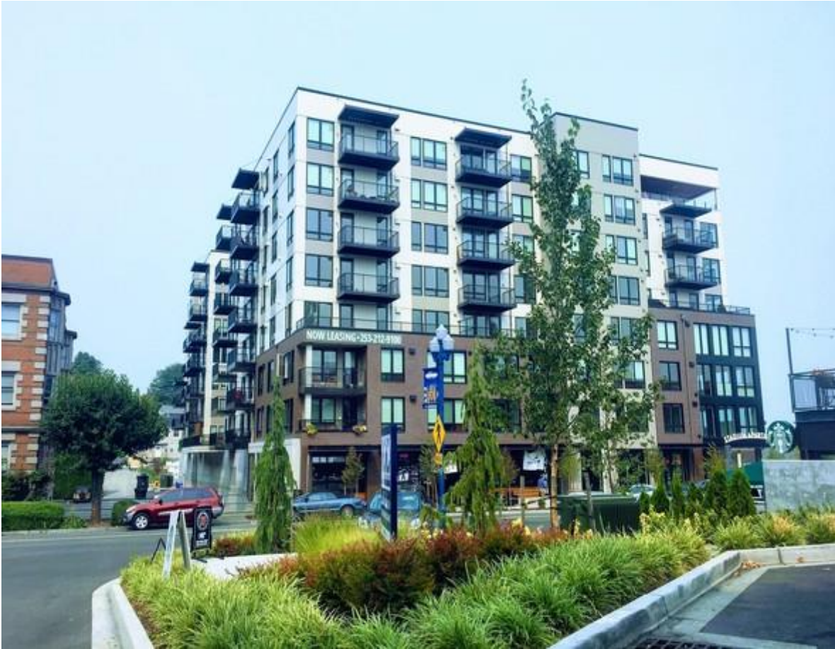
Completed Stadium Apartments Building on North G Street
